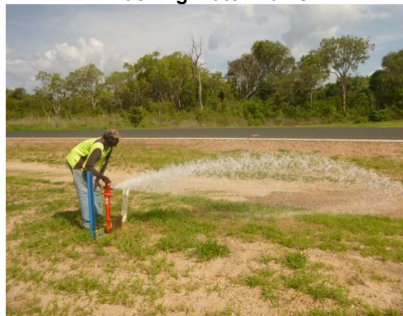
Flushing Water Mains
